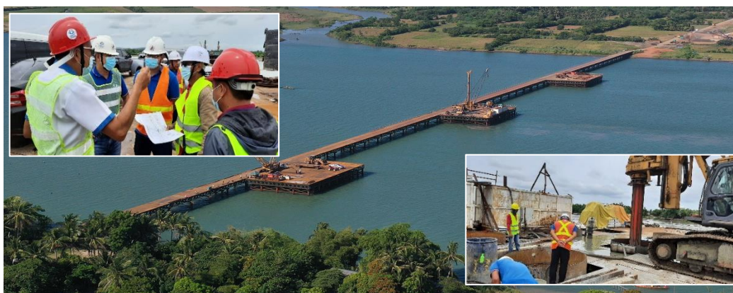
The RPMC visited the Camalaniugan bridge project in May 18, 2022. The construction of steel trestle (temporary bridge) and pier platforms and installation of 53 bored piles were completed. Boring is on-going in pier 20 using a 280-type rotary drill.
