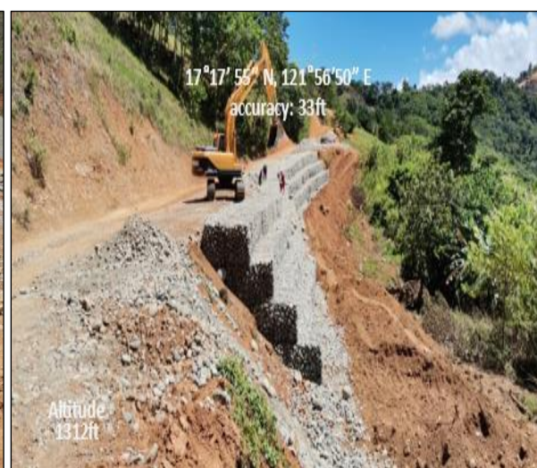
Slope Protection Along Access Road Extension 1
