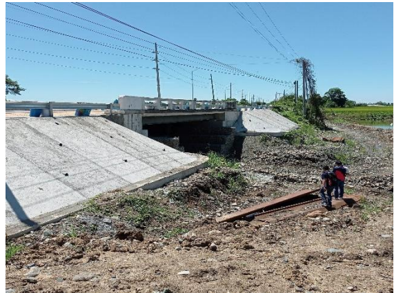
Repair Maintenance of Slope Protection along Daang Maharlika K0437+220-K0437+280, Cabagan, Isabela
