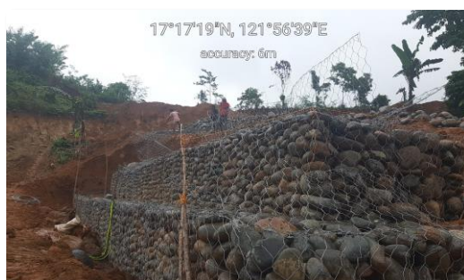
Gabion Works at Access Road 1 to Diversion Tunnel Outlet of the TRMP
