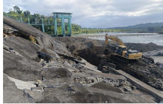
Damaged section of the Dummun River Diversion Dam and the on-going coffer damming activities as part of the rehabilitation works
