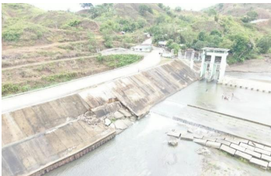
Damaged section of the Dummun River Diversion Dam and the on-going coffer damming activities as part of the rehabilitation works
