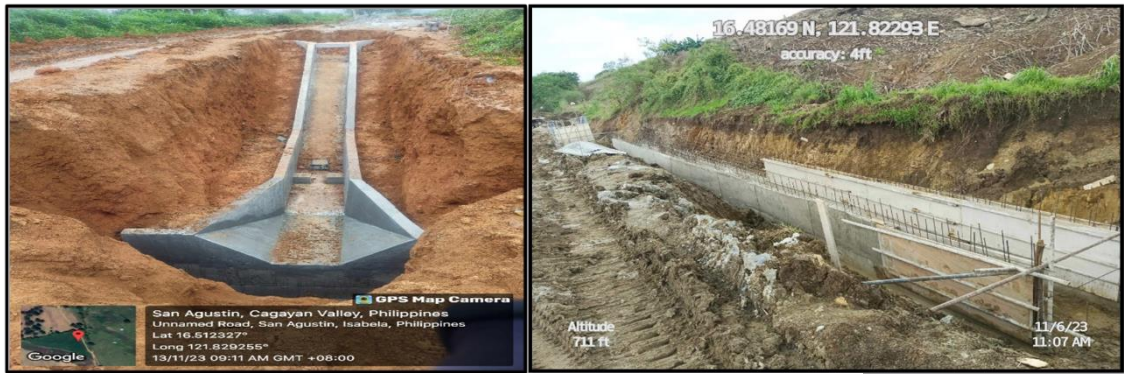
Ongoing construction of rectangular inclined drop and closed conduit barrel
