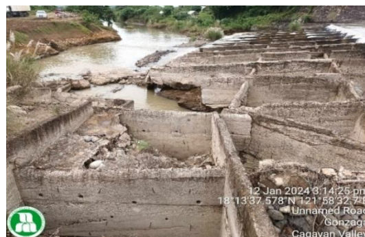
Damaged section and ongoing rehabilitation of the Nagbabacalan Diversion Dam in Gonzaga, Cagayan
