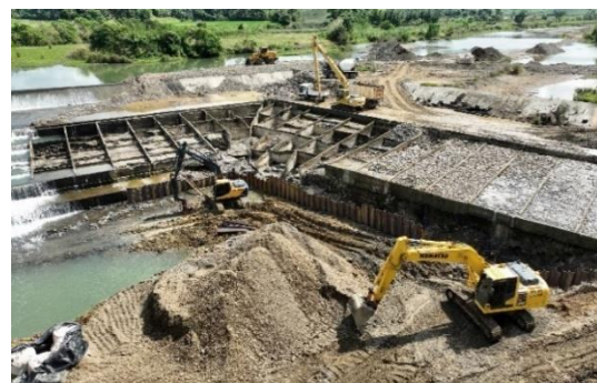
Damaged section and ongoing rehabilitation of the Nagbabacalan Diversion Dam in Gonzaga, Cagayan
