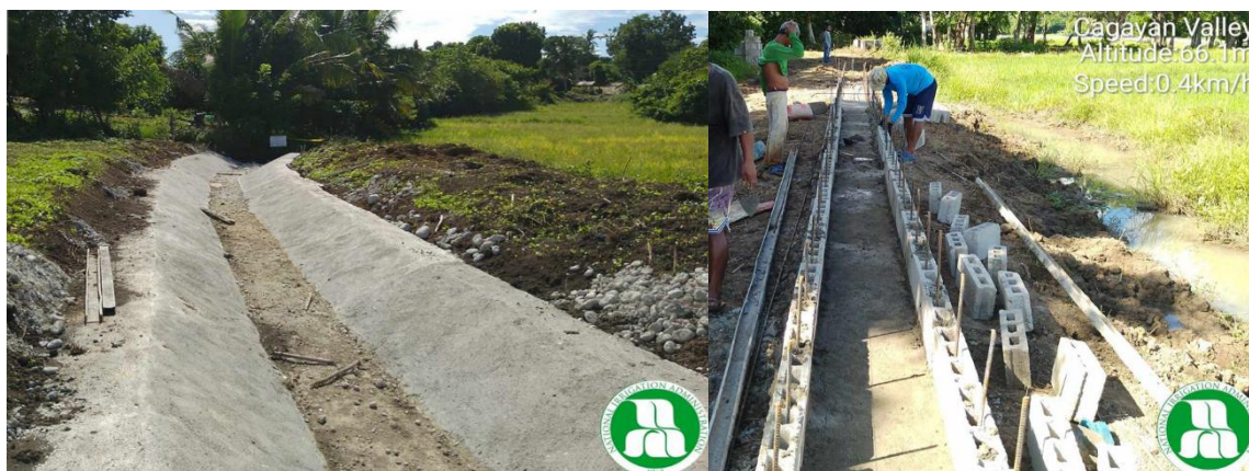
Ongoing construction of canal lining at km 13 main canal and CHB lining at Lateral A
